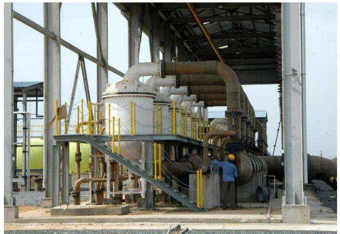
Pre-treatment Cartridge Filters
